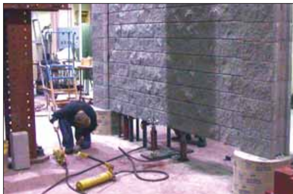
Assembled block wall with hydraulic jacks under the panel span for uplift test.
